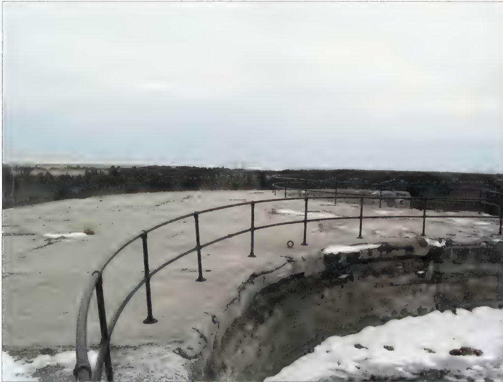
Figure 5.61. Recently installed contemporary safety railing, Battery Potter. Woven-wire may be either installed as infill panel, or the mesh applied with clamps to satisfy life-safety codes (Olmsted Center, January 2009).
